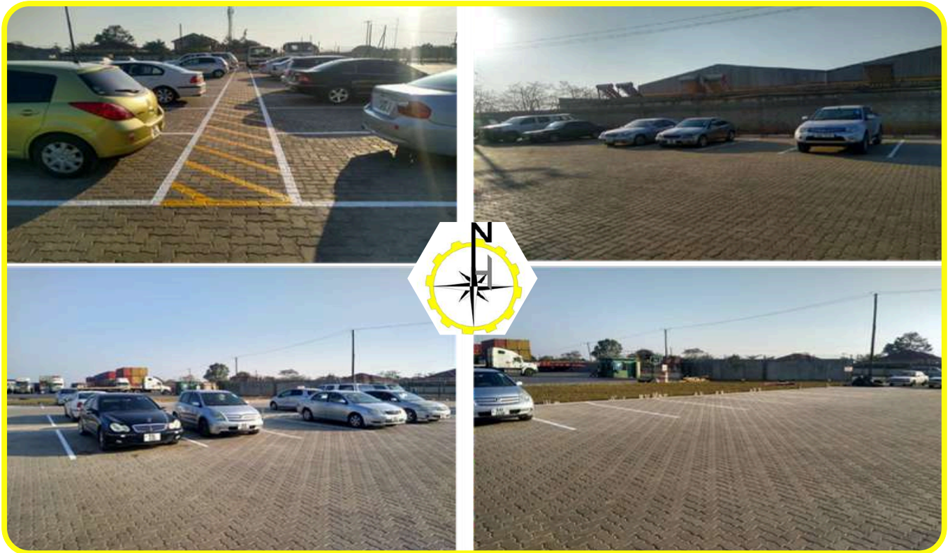
JJ Transport Zambia Limited – Car Park Markings, Bonaventure, Lusaka.
